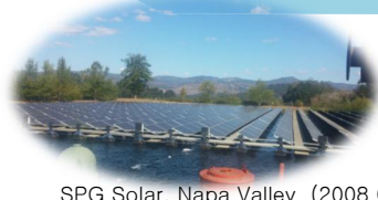
SPG Solar, Napa Valley (2008.06) 400kW 4.5 M$(1250만원/kW)
